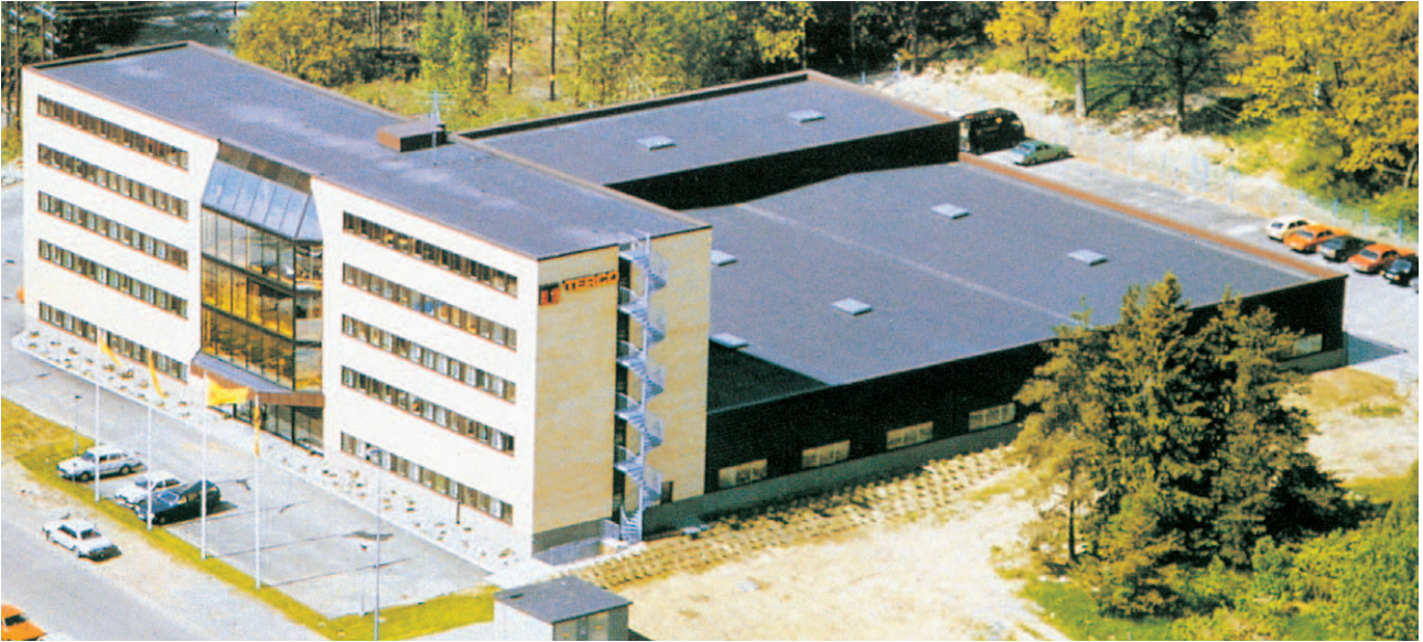
Terco headoffice and factory outside Stockholm, Sweden.
