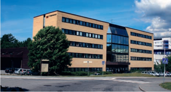
Terco headoffice and factory outside Stockholm, Sweden
