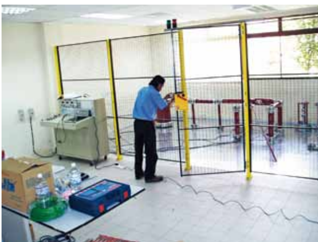
Installation of Safety Net
